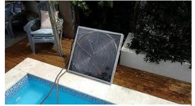
DIY solar pool heater Screenshot by Nicole Michael DIY is used under fair use https://www.youtube.com/watch?v=HdBCWR3z2D4
