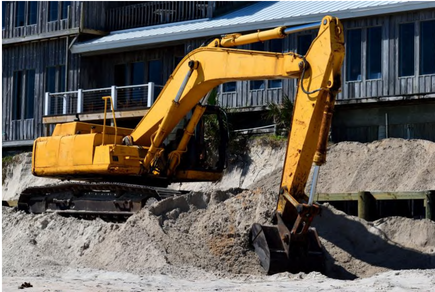
A backhoe working on beach erosion
