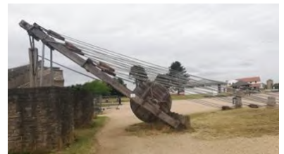
Image of a reconstructed Roman crane is used under fair use https://imperiumromanum.pl/en/cURIOSITIES/reconstructed-roman-crane/
