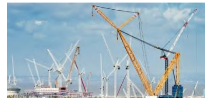
Image of Big Carl is used under fair use https://worldsteel.org/media/steel-stories/construction-building/worlds-biggest-crane-big-carl-is-steel-built-behemoth/
